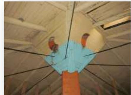
*Figure 70: Central bearing point for clear span of joists with panels displaying four cycles of the moon.*
